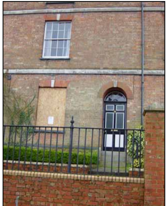
Hope Terrace, rubbed & gauged brickwork
