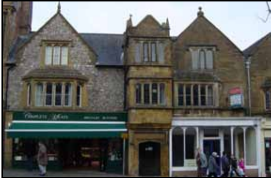
C16 coped gables, tall porches, mullioned windows
