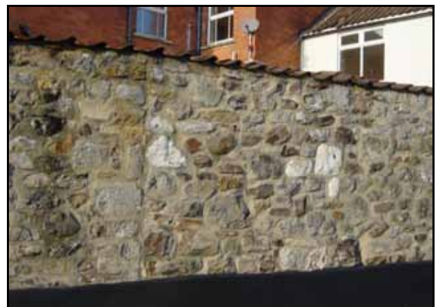
Rubble Chert wall, Silver Street
