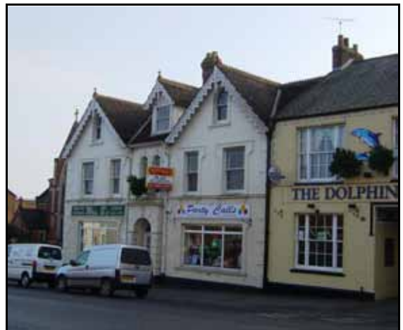
Eclectic Classical & Dutch details (top) & decorative details, barge boards, eared surrounds to marginal sashes, large dormer & rusticated entrance arch (above)
