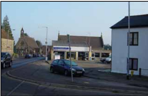
Eastern edge of conservation area: loss of enclosure
