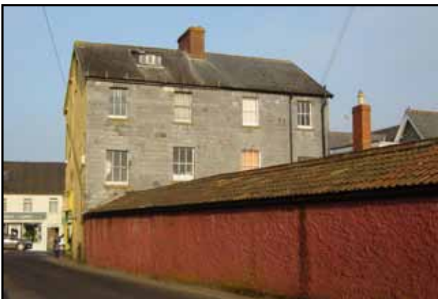
Slate hanging, rear of No. 28 Fore Street
