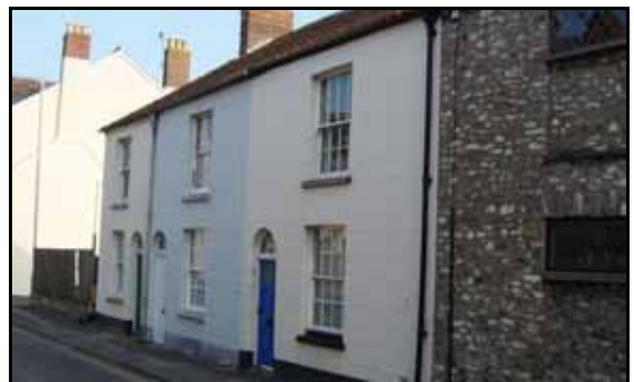
Classical vocabulary: grand gentry house (top) with tripartite window, cornice and expressed keystones; early C19 suave details (second from top) with larger first floor windows; rendered front (third) with careful window to wall proportions, paired doorcase & 8/8 sashes; rhythm of windows & doors (fourth) with radial fanlights
