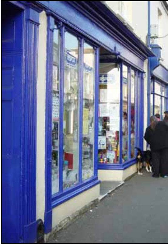
C19 timber shop front with moulded fascia, reeded pilasters, thin mullions & inset doorway
