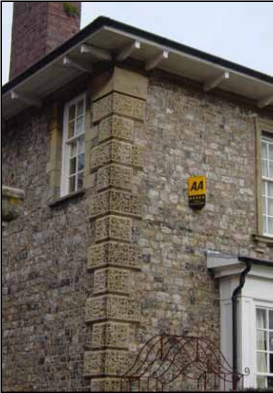
Mid C19, vermiculated quoins, careful use of quality materials, surrounds to sash windows & projecting, bracketed eaves
