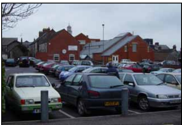
Modern buildings in Church St (top) & car parks (above)
